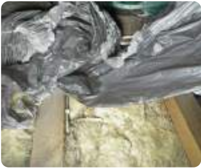
Photo 108 Roof void with debris and plastic sheeting; no visible defects.
