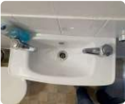
Photo 313 WC 1st Floor
