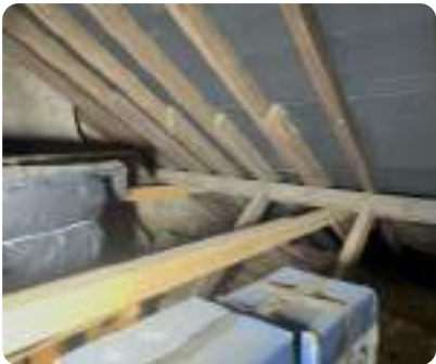
Photo 102 Roof void showing timber rafters and insulation; no visible defects.
