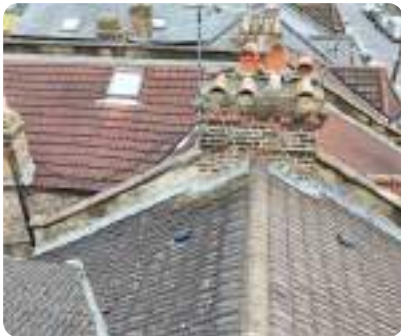
Photo 8 Chimney stack on the rear elevation; no visible defects.
