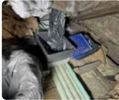
Photo 93 Roof void observed with stored items and insulation material; no visible defects.
