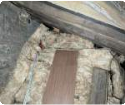
Photo 106 Roof void with visible insulation and timber; no visible defects.
