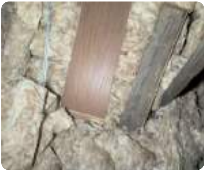
Photo 107 Roof void showing insulation material and wooden beams; no visible defects.
