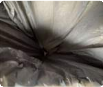
Photo 109 Roof void within the property showing plastic sheeting; no visible defects.
