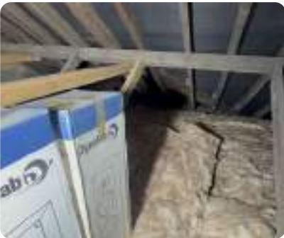
Photo 103 Roof void observed with exposed timber rafters and insulation; no visible defects.
