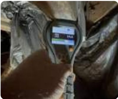
Photo 110 Roof void showing moisture meter reading of 14.4; no visible defects.
