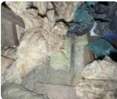
Photo 98 Roof void showcasing insulation material and cluttered items; no visible defects.
