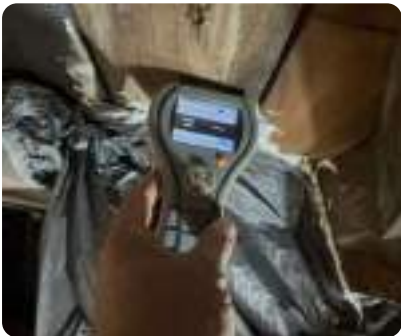
Photo 113 Roof void area showing moisture meter in use; no visible defects.
