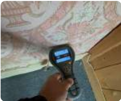
Photo 223 Bedroom 3 - Wall behind the bath in bedroom 3
