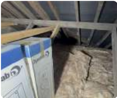
Photo 103 Roof void observed with exposed timber rafters and insulation; no visible defects.
