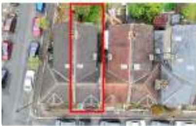
Photo 2 Main roof viewed from above
