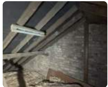
Photo 100 Roof void showing timber framing and insulation; no visible defects.
