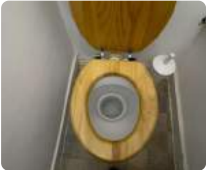
Photo 512 WC Ground Floor
