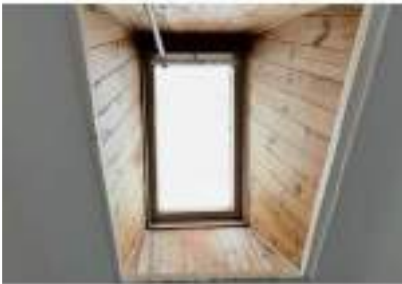
Photo 315 Hallway - Velux window no evidence of active leaks.
