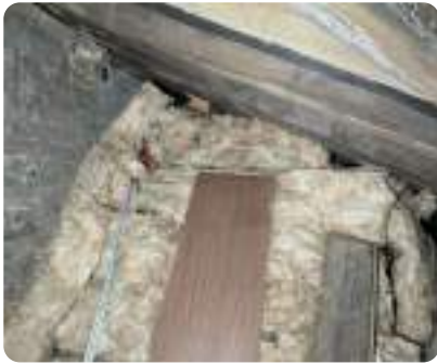
Photo 106 Roof void with visible insulation and timber; no visible defects.
