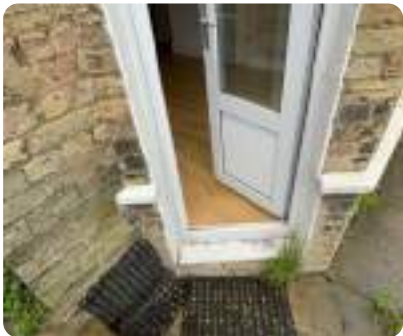
Photo 72 External Walls - This rear bay has been structurally altered with a new door opening.
