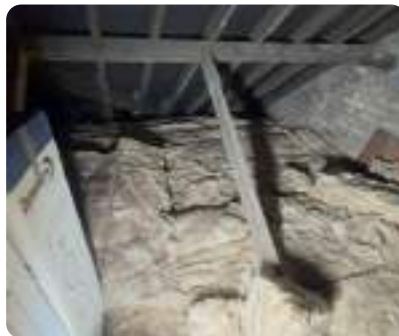
Photo 99 Attic space showing insulation material; no visible defects.
