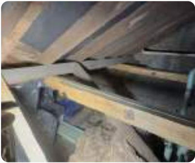
Photo 105 Roof void showing timber framing and insulation materials; no visible defects.
