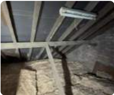
Photo 101 Roof void showing timber rafters; no visible defects.
