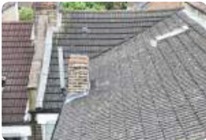
Photo 6 Chimney stack on the main roof; no visible defects.
