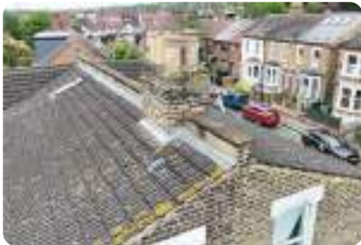
Photo 3 Rear elevation main roof in clay tiles; no visible defects.
