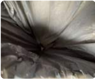
Photo 109 Roof void within the property showing plastic sheeting; no visible defects.
